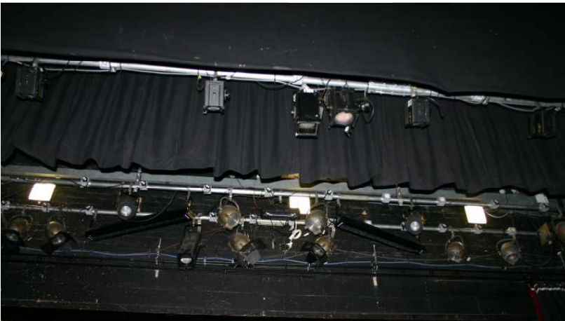
Looking towards auditorium LX Bars in this picture: 1, 2, 3
